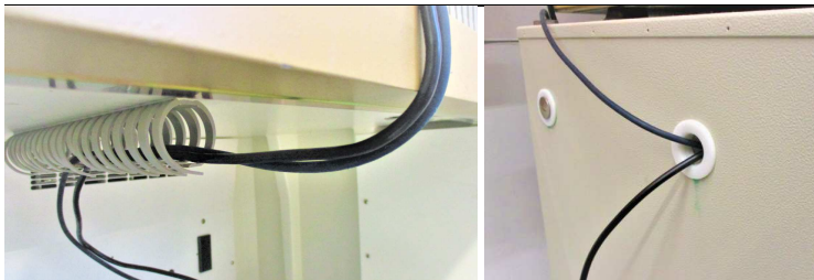
Figure 3: Routing of Power elongation and USB cable.
